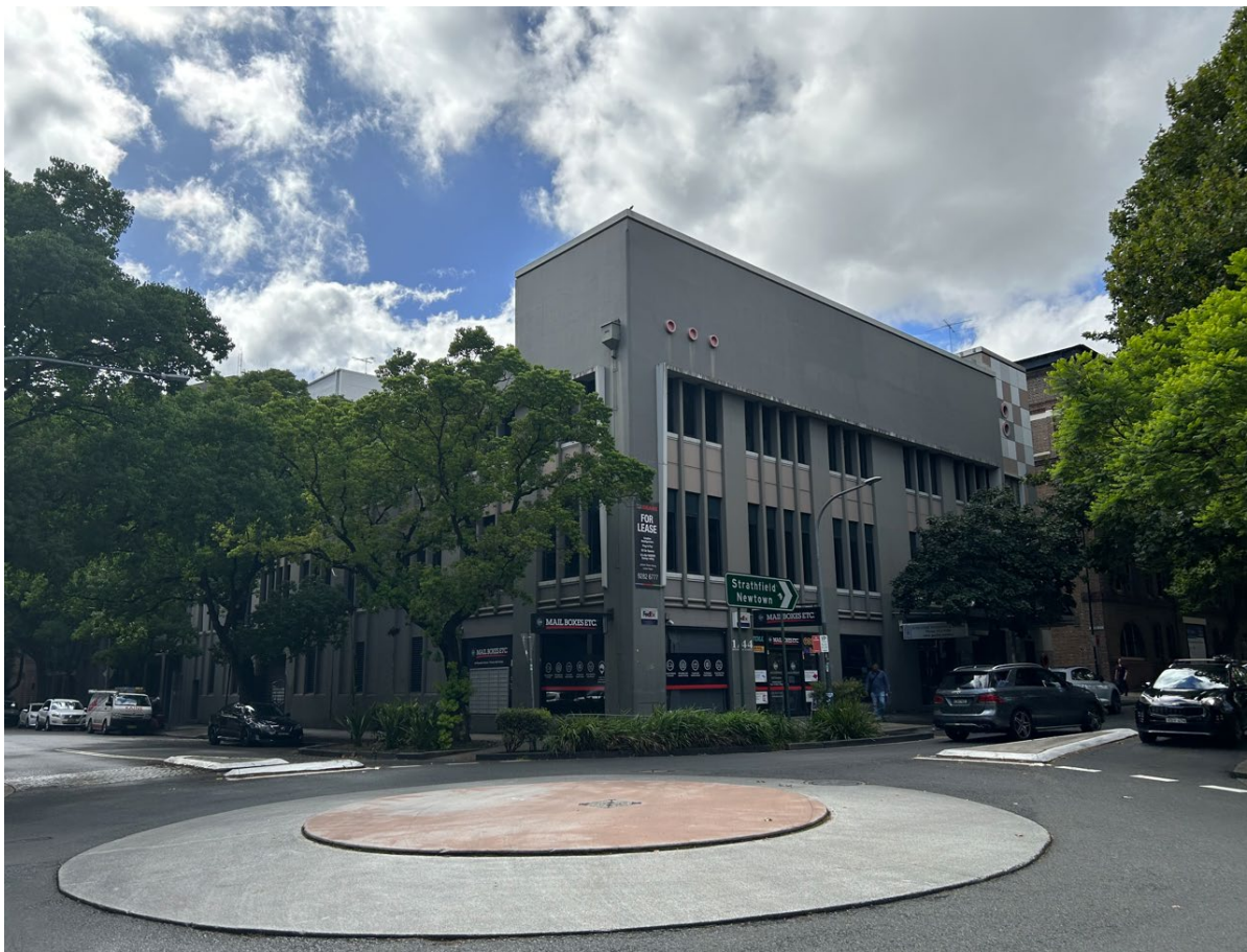
Subject site viewed from across intersection of Mountain Street and Small Street, facing southeast
